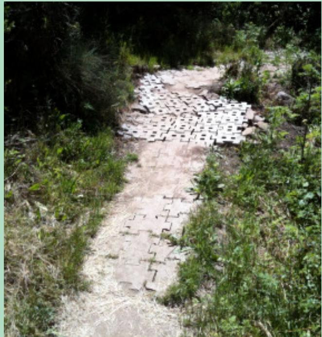
The new blocks joined those previously installed, and will enable water to flow through in the winter without creating more mud on the trail.
